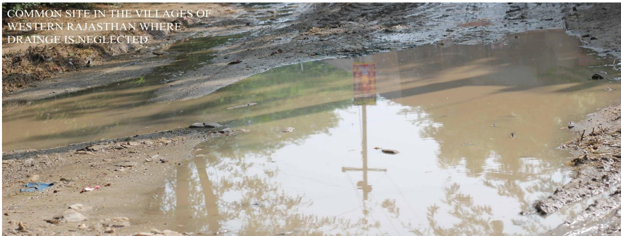
Photo.12. open drainage in village Inderpura, Didwana.
